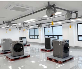
▲ Refurbishment Center (Cleaning Room)
